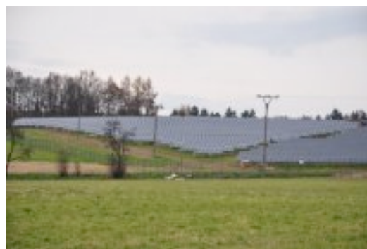
Image. : Solarpark in Komarice ( Czech Reupublic ) , approx. 847 MW Power
